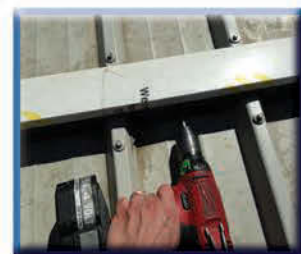
Roof external profiles
